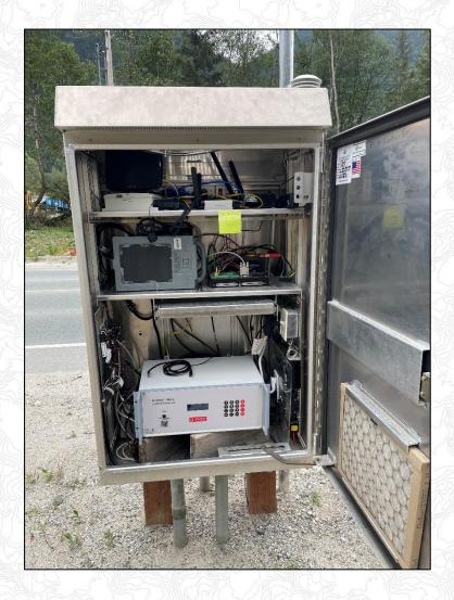
In my first two roles with DOT&PF, I was trained in maintenance and calibration of roadside traffic sensors. The continual operation of these sensors was essential to our traffic monitoring program and necessary for federal reporting.
